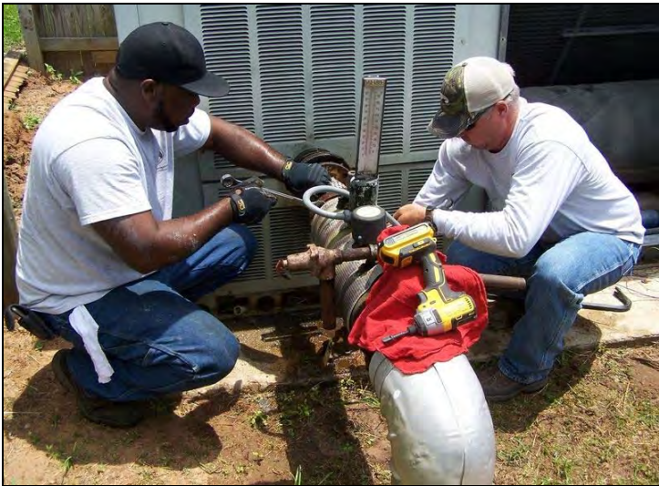
Building Mechanical Repairs and Improvements
