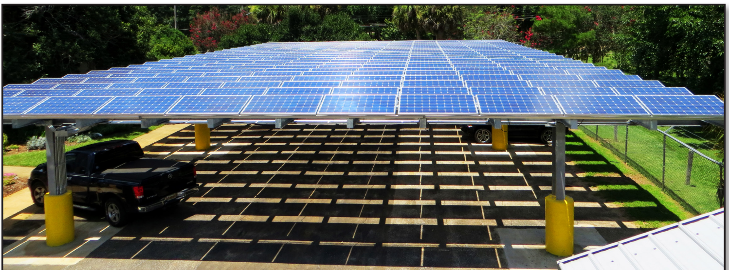
Leon County Net-Zero Facility
