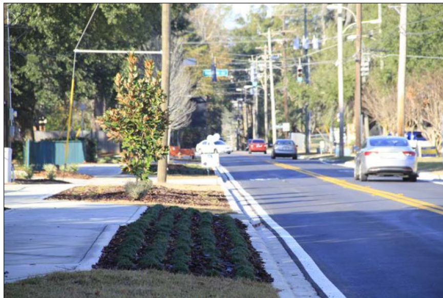
Roads Pavement Markings
