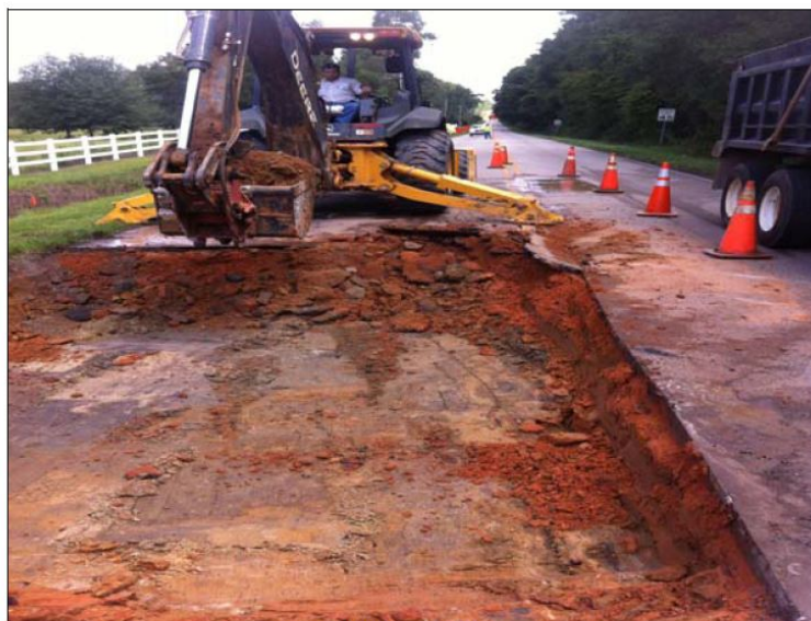
Asphalt Road Maintenance
