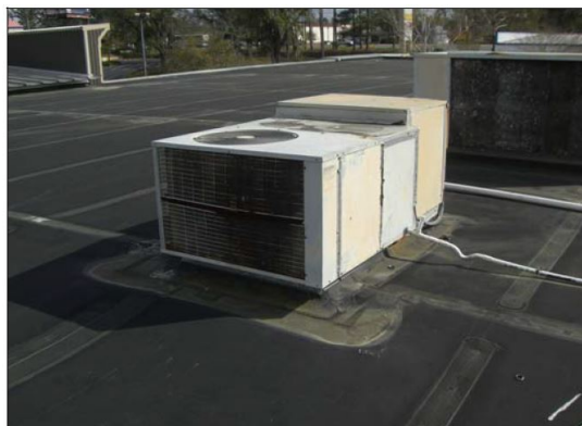
Building Roofing Repairs and Replacement
