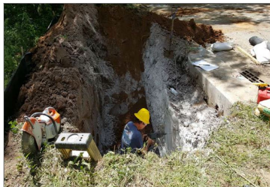
Stormwater Infrastructure Preventive Maintenance
