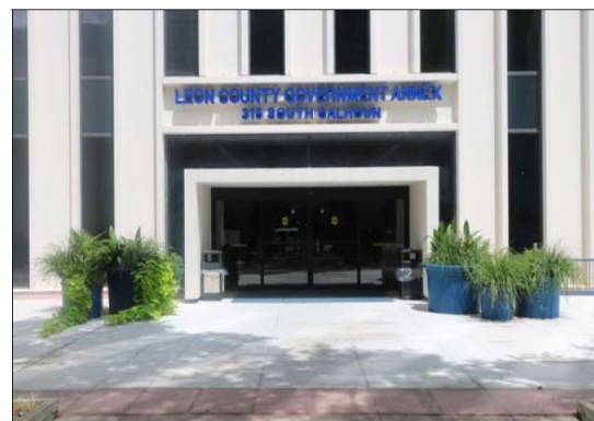
Leon County Government Annex Building
