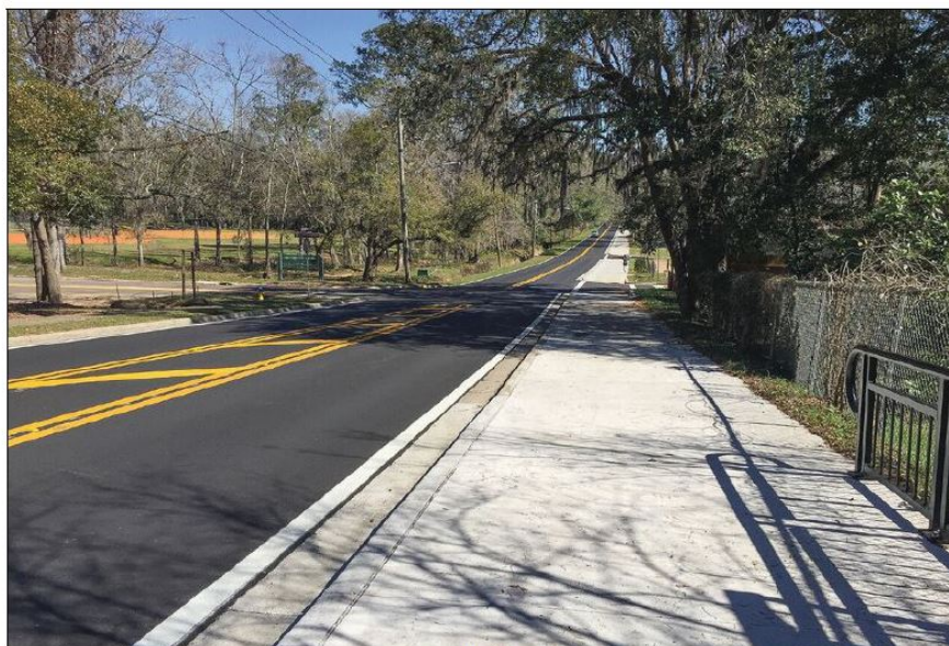
Local Road Resurfacing
