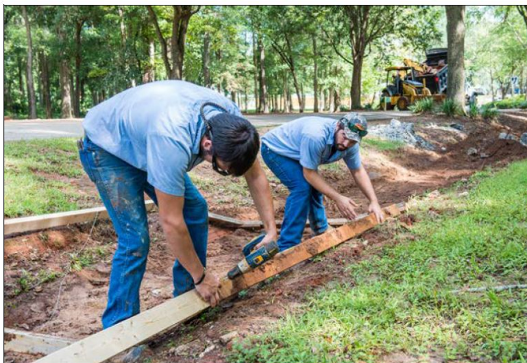
Construction of sidewalk for Community Safety & Mobility
