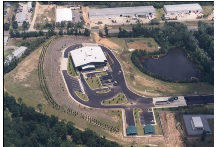
Leon County Transfer Station
