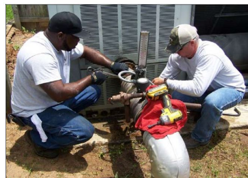
Building Mechanical Repairs and Improvements
