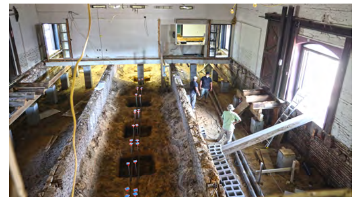
Renovations at Amtrak building
