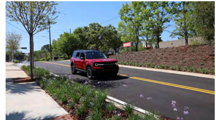
Major infrastructure improvements on Magnolia Drive
