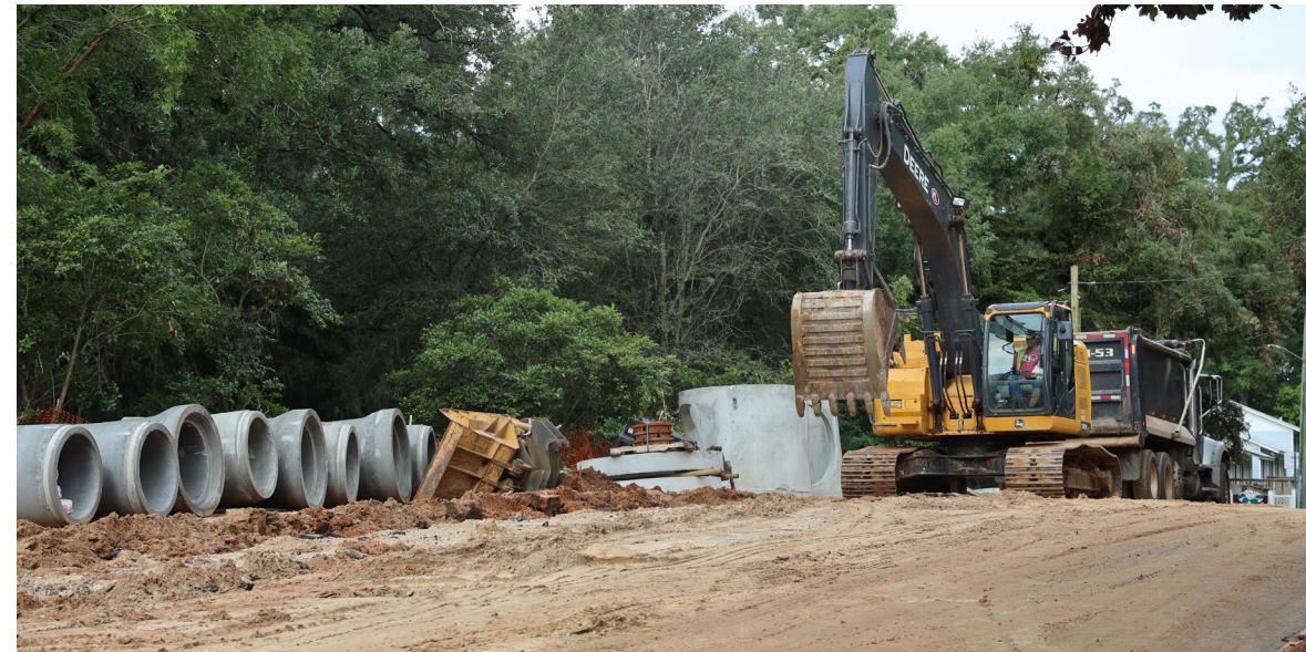
Major Infrastructure Improvements on S. Magnolia Drive
