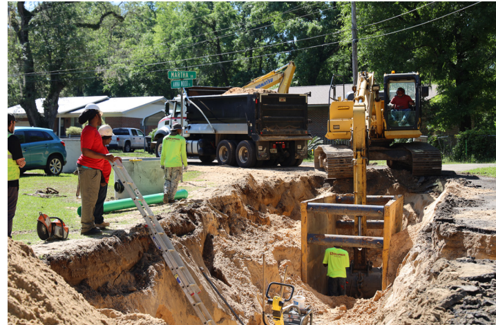
Annawood septic-to-sewer upgrades
