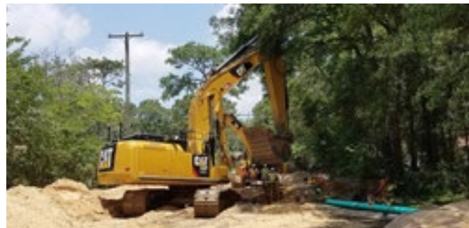
Woodside Heights sewer line construction
