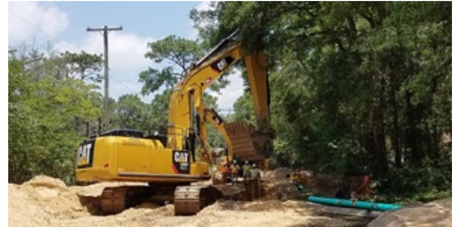
Woodside Heights sewer line construction
