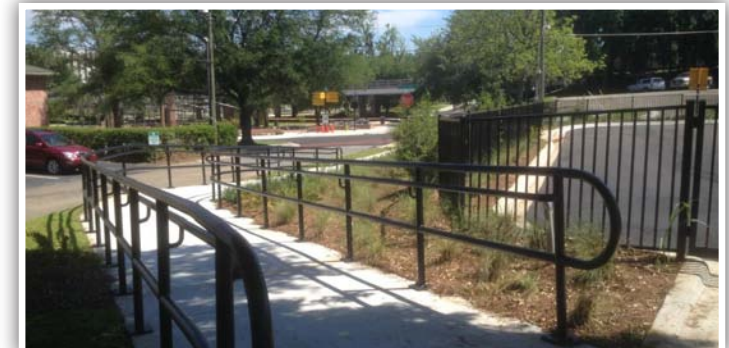
Sidewalk Improvements for Cascades Park
