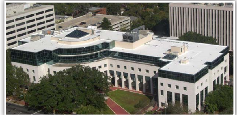
Leon County Courthouse Rooftop
