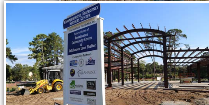
Construction of Comprehensive Emergency Services Center
