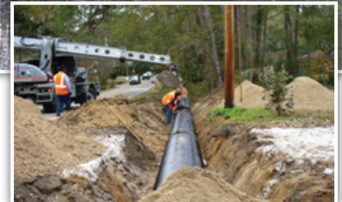
Stormwater crews installing driveway culverts
