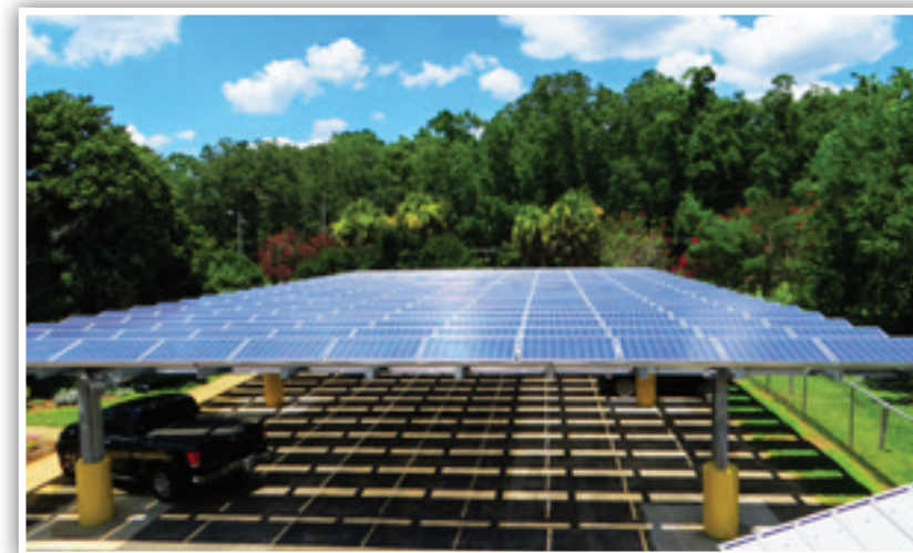
Cooperative Extension Net-Zero Facility
