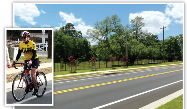
Buck Lake Road Reconstruction Project
