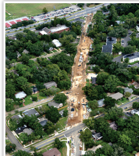
Franklin Boulevard Construction
