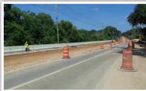
Buck Lake Road Reconstruction - Phase III
