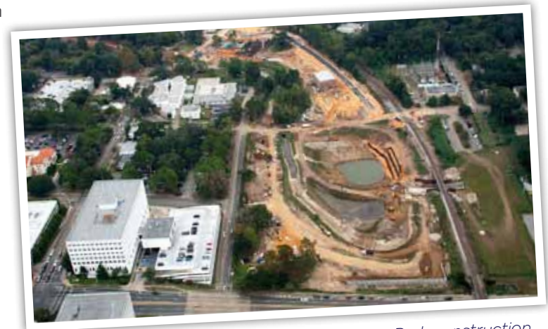
Aerial photo of Capital Cascades Park construction
