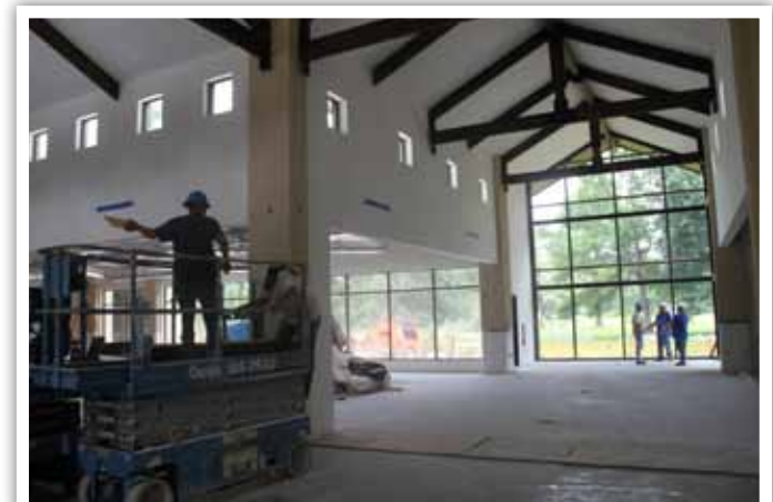
Eastside Branch Library Construction In Progress
