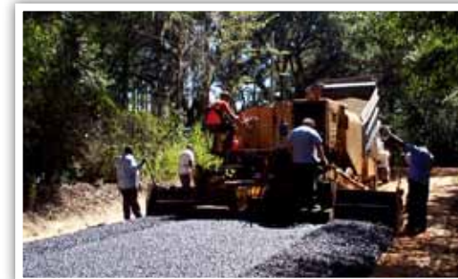
Road Work In Progress
